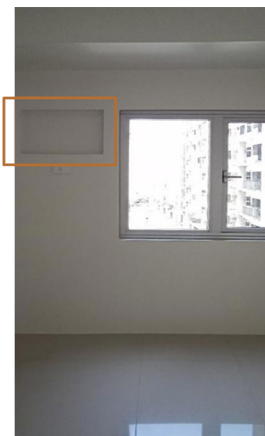
400mm x 600mm Block-out with cover for WACU
