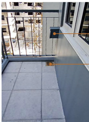
NEMA 3R Circuit Breaker for ACCU
