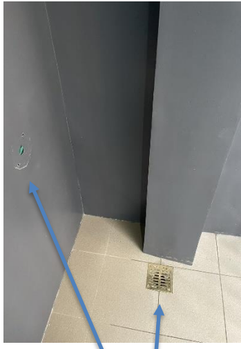
Balcony drain and provision for Circuit Breaker of ACCU
