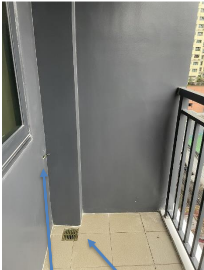
Balcony drain and provision for Circuit Breaker of ACCU
