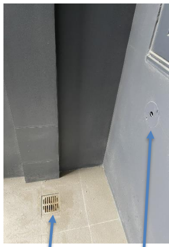
Balcony drain Provision for Circuit Breaker of ACCU
