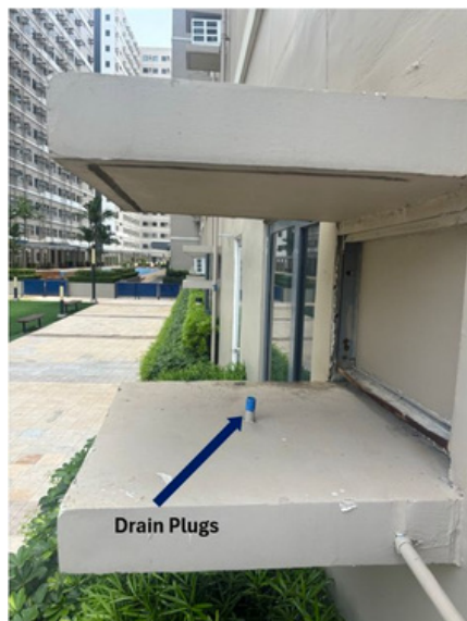
Figure A-2. ACU Drain Plugs
