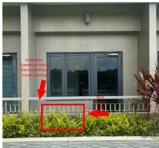
Figure B-2. Outdoor Unit Position with Pipe Sleeves
