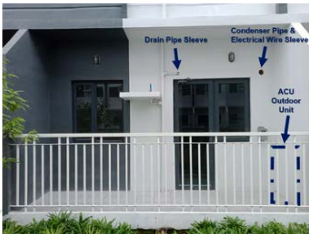
Figure B-2. Outdoor Unit Position with Pipe Sleeves
