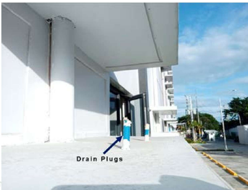
Figure A-2. ACU Drain Plugs
